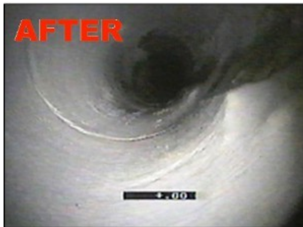
This 6" inch pipe had heavy build up where an 1-1/2" + of pipe diameter was lost on each side
